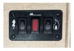
If you can't track down the problem, you can always switch to propane. Just turn off the left switch and turn on the right switch.
